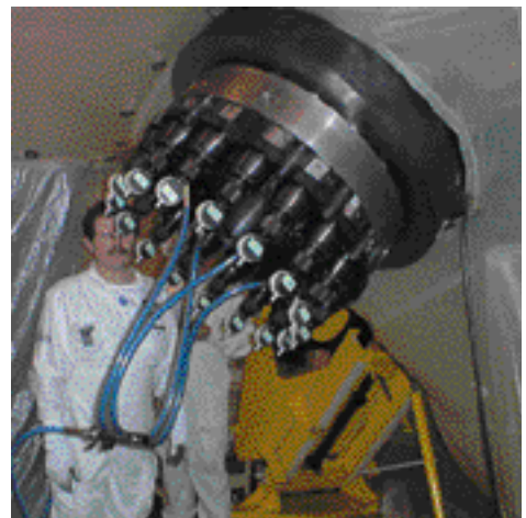
On-site intervention, tightening the man hole hatch on the primary cooling system of a steam generator.
